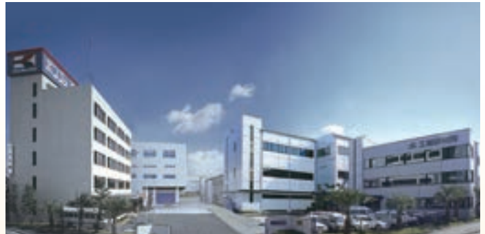
Head office and factory
